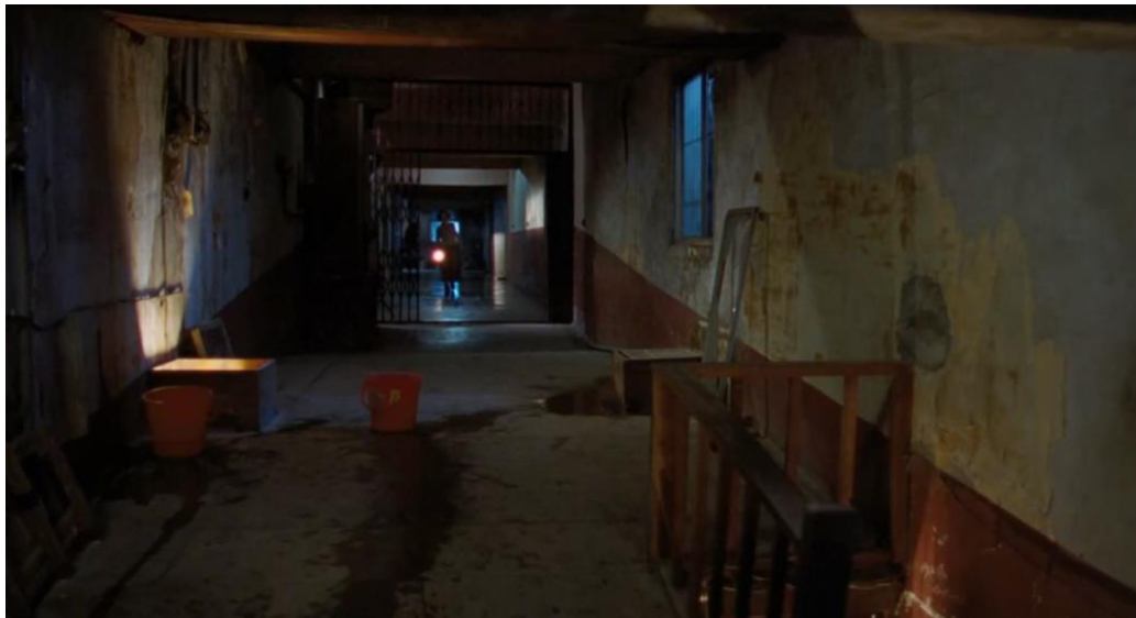
Figure 15: Peeling paint and leaking ceiling in Goodbye, Dragon Inn (Ming-liang, 2003)
