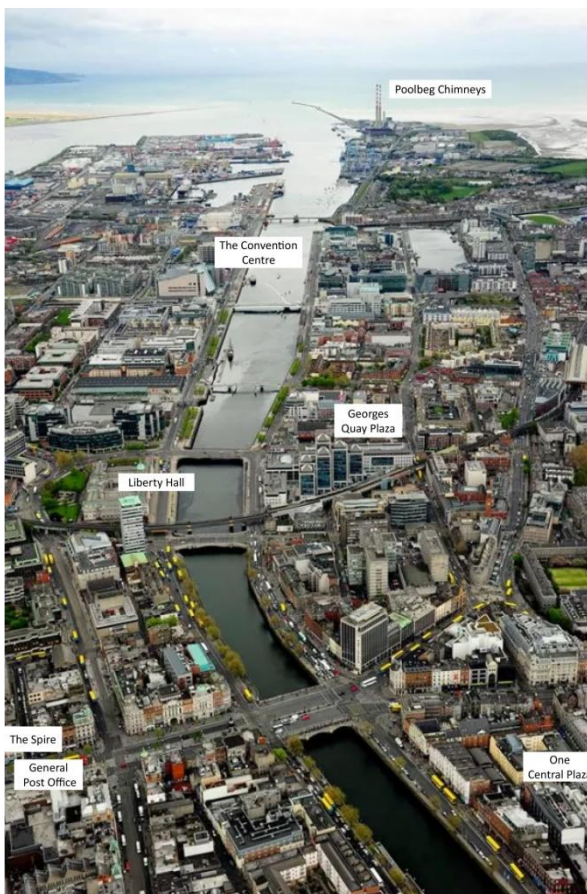
Figure 12. Aerial view of Dublin City with a selection of buildings from Babel labelled by the author
