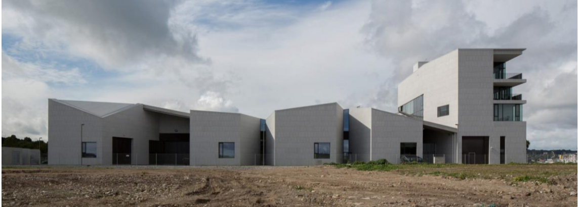
Figure 2. The Beaufort Maritime and Energy Research Laboratory UCC façade
