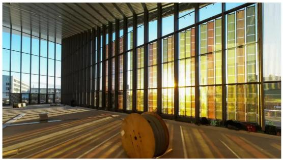
Fig. 26 Grätzel cells installed at the SwissTech Convention Centre (credit: Alain Herzog)
