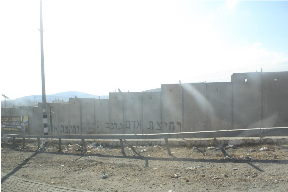
Figure 8, Jamie Howard, West bank border wall with Hebrew graffiti, 25 September 2023.
