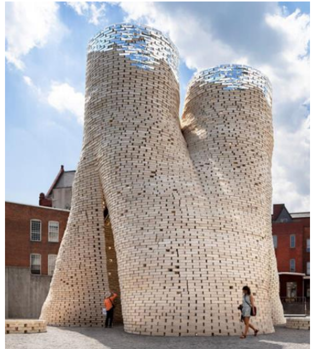
Figure 14 - Mycelium-Grown Bio-Bricks / Evocative Design & The Living. Image Courtesy of The Living 1
